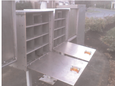
One piece, 3/16" aluminum door with postal lock repositioned and an H-4800r kit installed.
